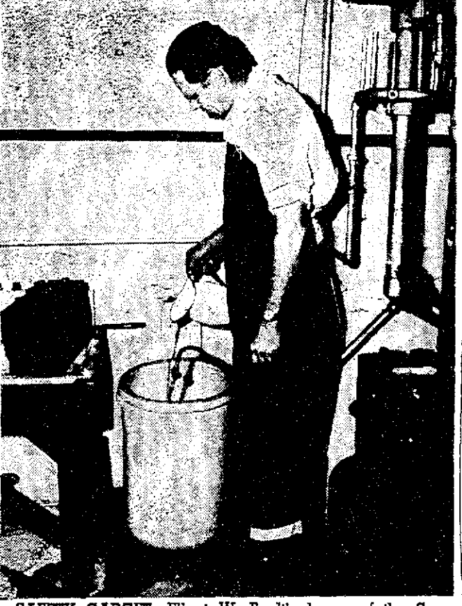
SAFETY GADGET —Elbert W. Boultinghouse of the San Antonio General Depot pours water into crock prior to turning on air and adding sulfuric acid. His gadget, which insures safe, comfortable working conditions and for which he was awarded a cash prize, protrudes from the crock. Worker need not stand over acid fumes now.
