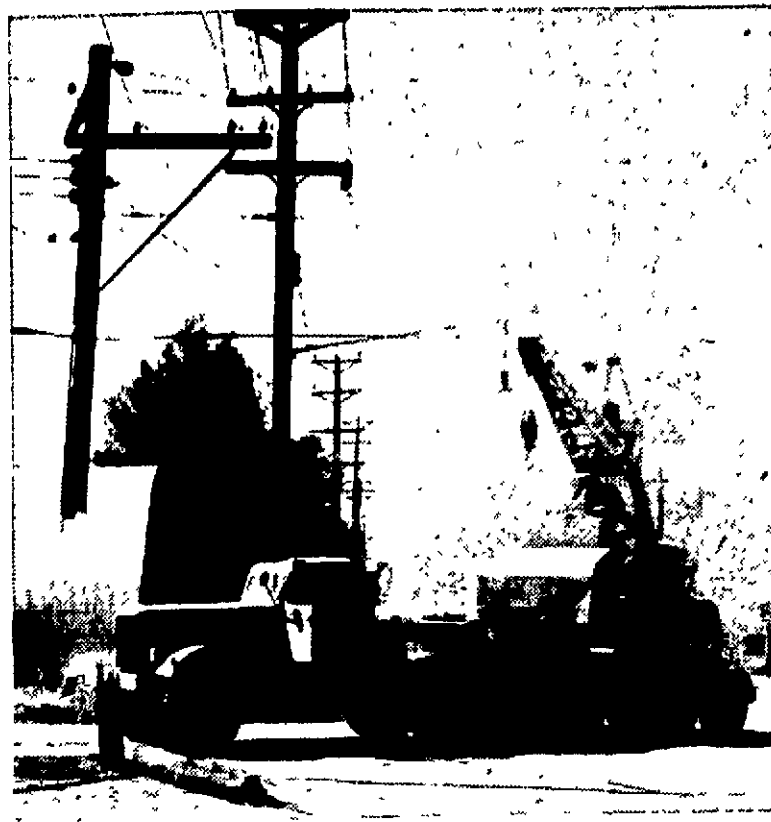
CRANE CLIPS UTILITY POLE —Claude Napier, Beaverdam, driver of a Lima Tank Depot tractor-trailer hauling a crane, carefully avoided hitting a street light at the corner of Fourth-st and St. Johns-av early Wednesday afternoon. While he was making sure the crane boom didn't damage the street light, however, it swung wide with the trailer and clipped out a 10-foot section from a utility pole on the southeast corner. High tension wires supported by the pole flipped up in the air and burned off a dozen telephone lines on the north side of Fourth-st. Napier was en route to the tank depot storage area a mile south of the city on the St. Johns-rd. The mishap occurred as he was eastbound, turning south onto St. Johns-rd.
