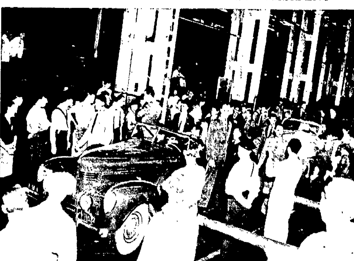
Halting work briefly, workmen at the Chrysler tank arsenal in Detroit, greet President Roosevelt as he drives thru the great factory on a tour of inspection which took him to armament plants across the country.
