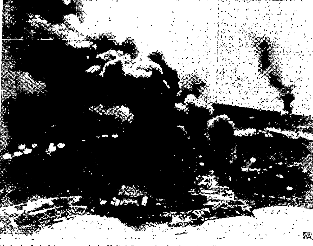
This is the first picture to reach the United States showing how the valiant Dutch scorched the earth as Japanese invaders poured into the Netherlands East Indies. Here millions in oil and oil installations go up in smoke at Balikpapan on the east coast of Borneo.
