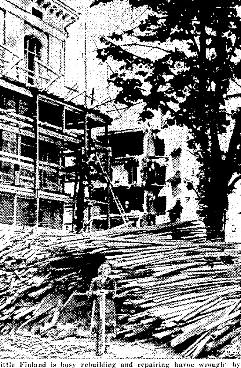
Little Finland is busy rebuilding and repairing havoc wrought by the military claws of the Russian bear. This photo shows a building in Helsinki encased in scaffolds as bomb damage is repaired. In background is another wrecked structure. Women, like the one in the foreground, are helping with construction work.
