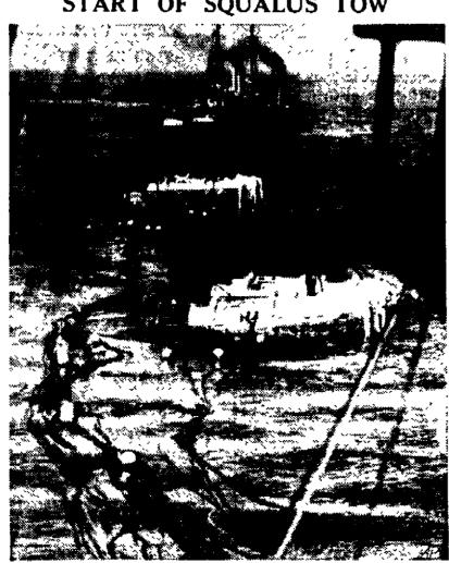
Looking from the salvage ship Falcon can be seen the six pontoons that came to the top when the submarine Squalus was lifted off the bed of the ocean 80 feet, off Portsmouth, N. H. Many air lines from the Falcon pumped air into the pontoons. The Wandank, in background, is slow towing the Squalus and Falcon to shallower waters.
