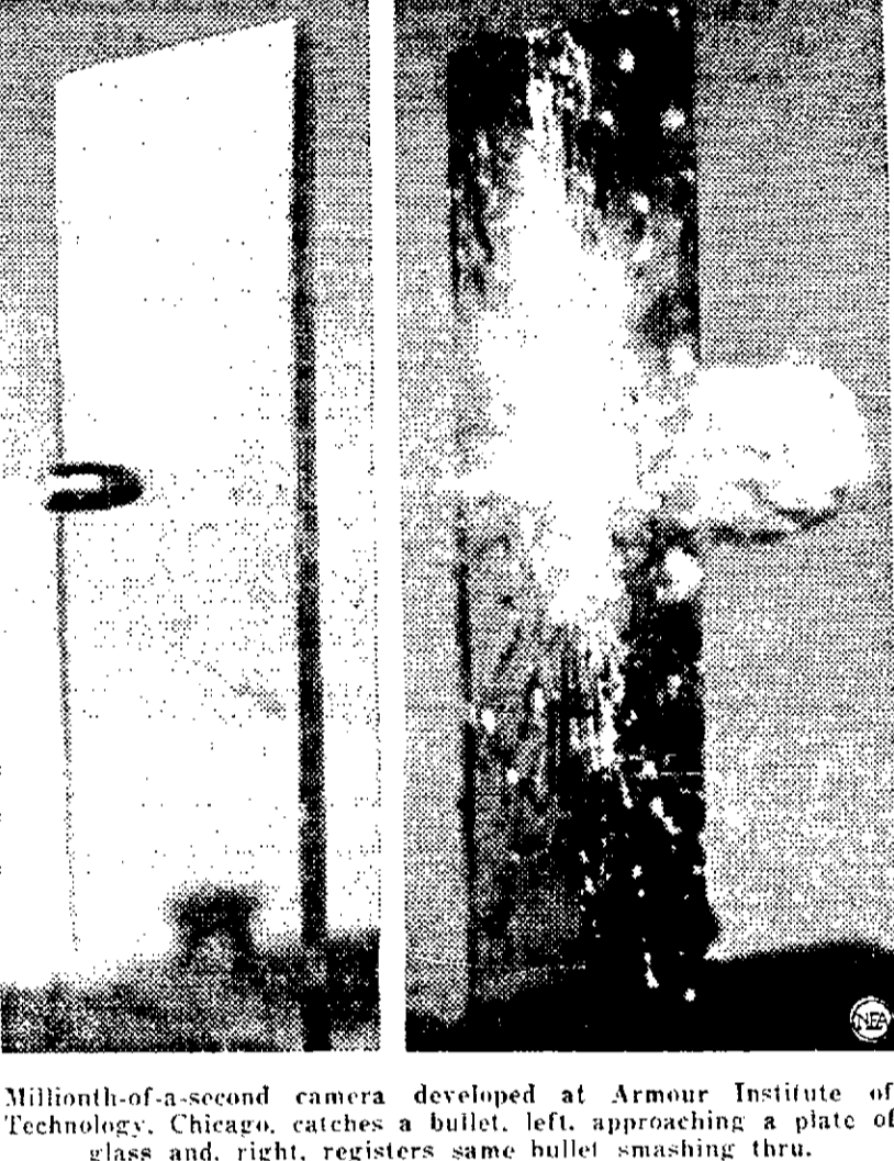
Millionth-of-a-second camera developed at Armour Institute of Technology, Chicago, catches a bullet...
